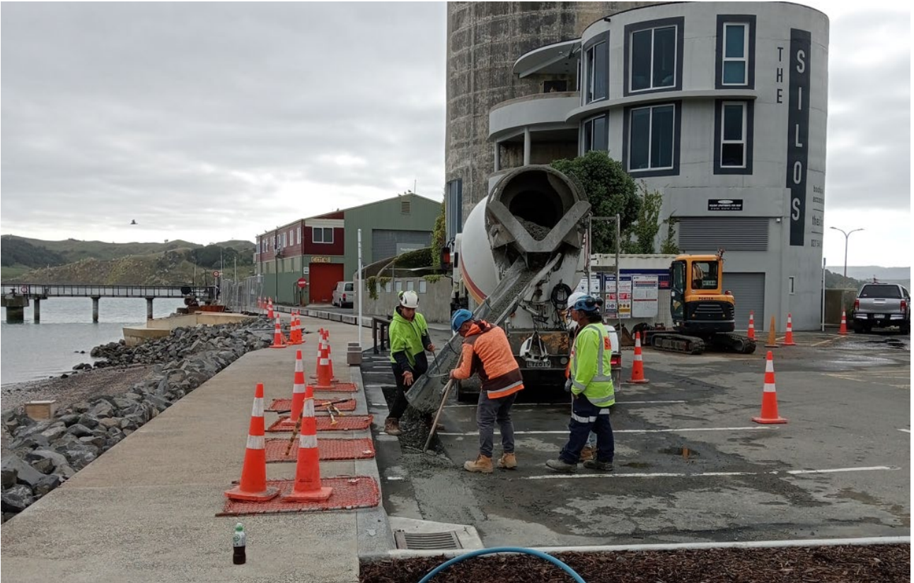
Pouring wheel stop footings before asphalt resurfacing
