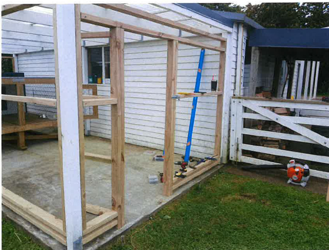
Enclosure being built
