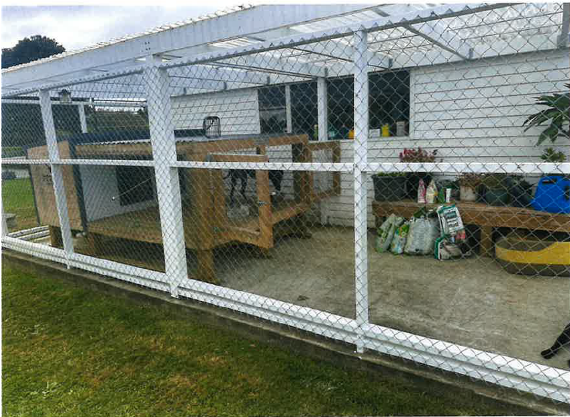
Completed Containment Area 2
