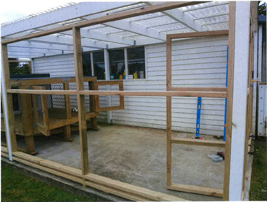
Enclosure being built including kennels
