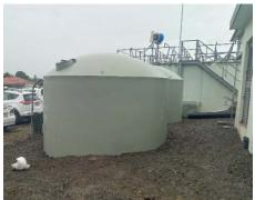
The run to waste storage tanks were secured in position ready for the pipework to commence.
