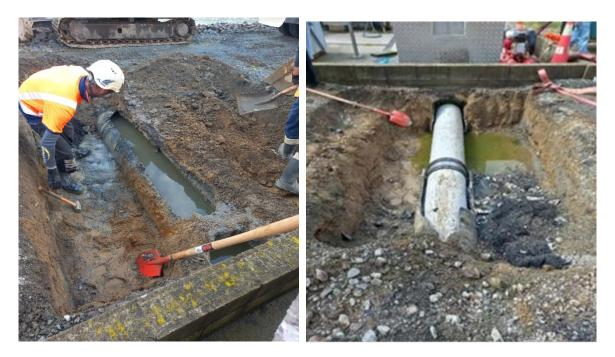
Figure 2 - Corrosion at the treatment pond inlet (L) and temporary fix of a length of this pipe (R)
