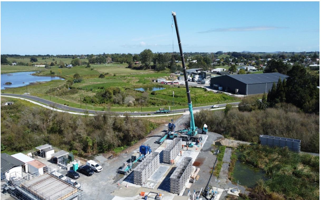
Te Kauwhata WWTP temporary Ultra filtration plant has been installed and commissioned by Spartan/Veolia and is now operational. Initial 2 test results show an improved treatment performance for suspended solids from  $>30\text{g/m}^3$  to  $3\text{g/m}^3$  and then  $1.6\text{g/m}^3$  against a measure of  $15\text{g/m}^3$ , which is a great result.
