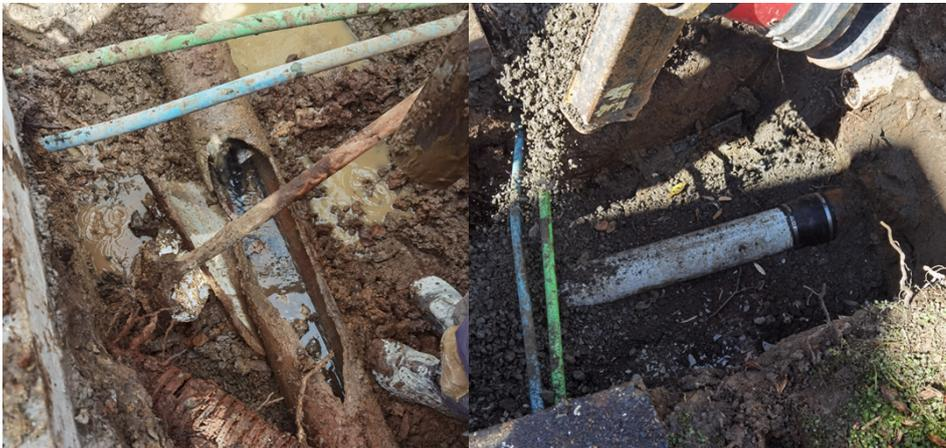
42 Wainui Rd, Raglan – 100mm WW main repair. The CCTV surveys picked up another job. A significant hole in the wall of the pipe was observed, which required action. The defective length of the pipe was removed and replaced.
