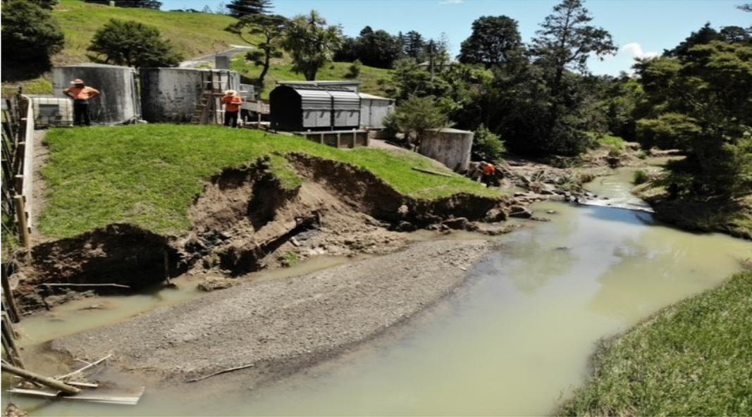
The portion of bank erosion upstream of the plant will be challenging to remediate due to the lack of access. The chlorine contact tank will be relocated to provide access to install “gabion baskets” to protect the bank from further erosion and support backfilling the bank. A new plastic tank will be installed in place of the removed old concrete tank. There is a minimal footprint available for this work. Costs have been provided to Waikato District Council for an insurance claim.
