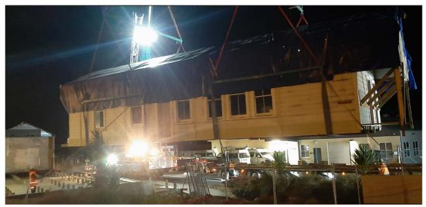
Lifting of damaged section on to permanent site.
