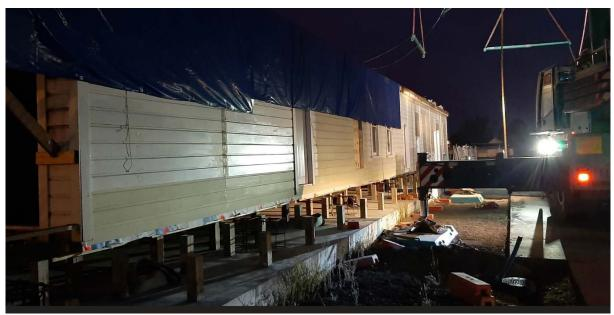
Damaged section being placed on piles in permanent location.
