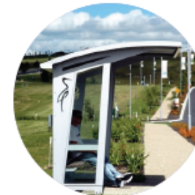
Upgraded bus shelters
