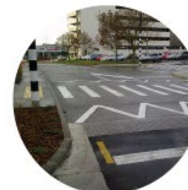
Raised pedestrian crossing
