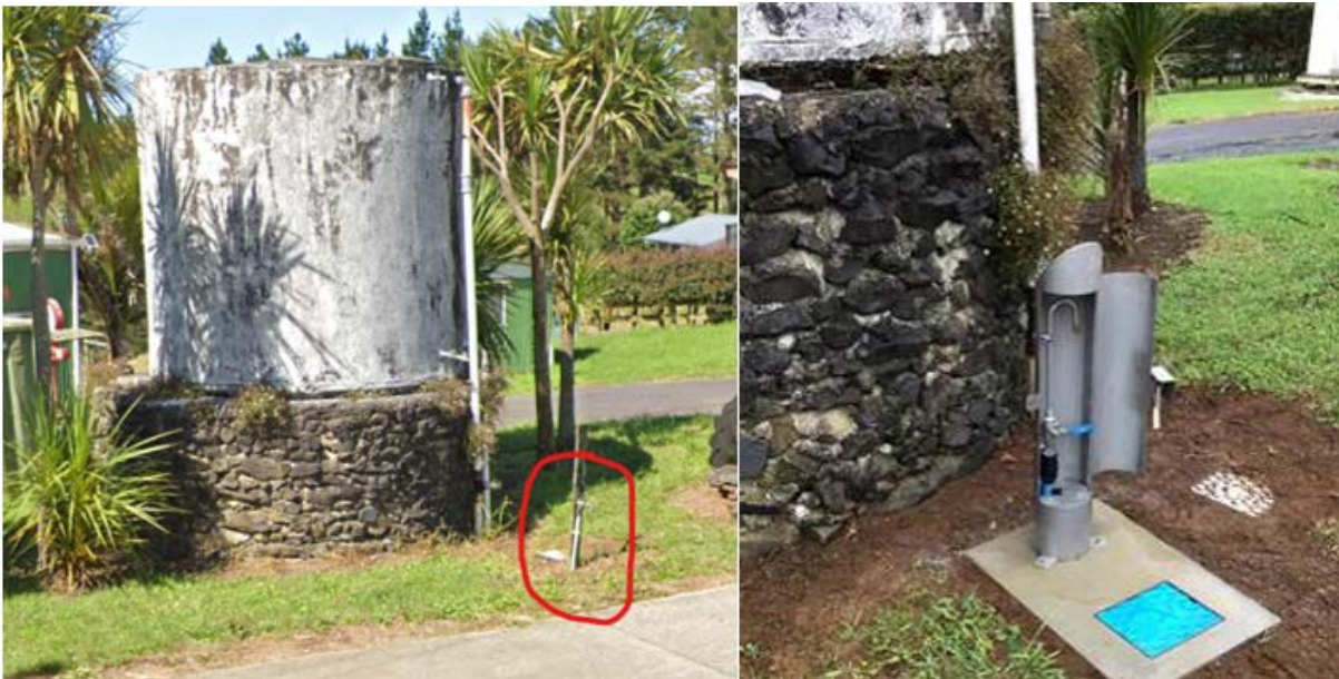
Figure 1. Garden tap replaced with hygienic sample bollard in Onewhero.
