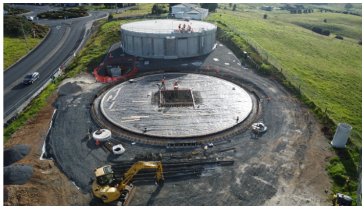
Te Kauwhata Reservoir 2- Tying the base slab reinforcing.
