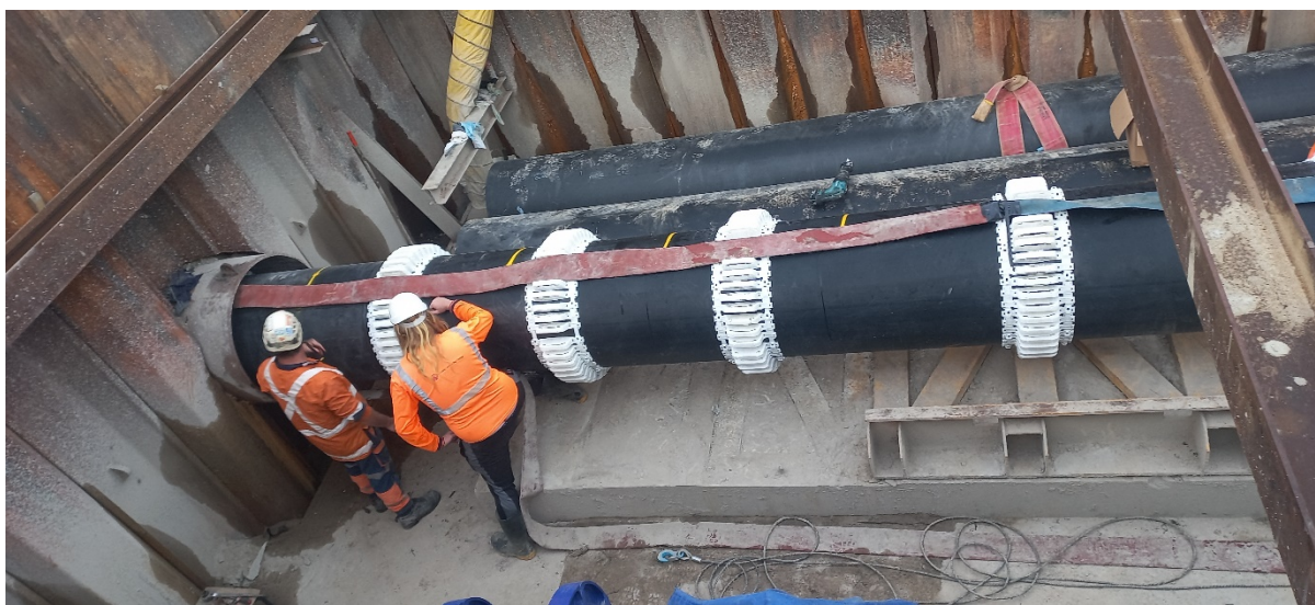
Ngāruawāhia Pipeline - The undertrack pipe being pulled into the casing
