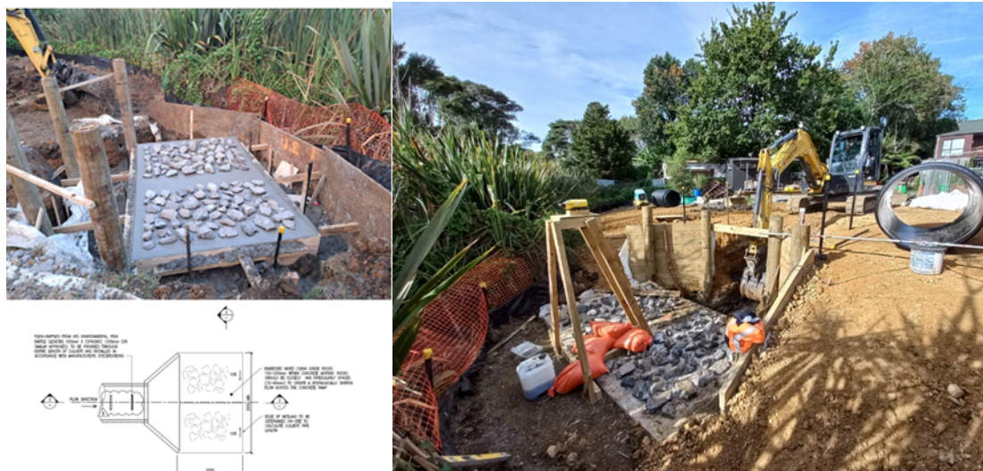
Cambrae Road Culvert Upgrade – Downstream headwall
