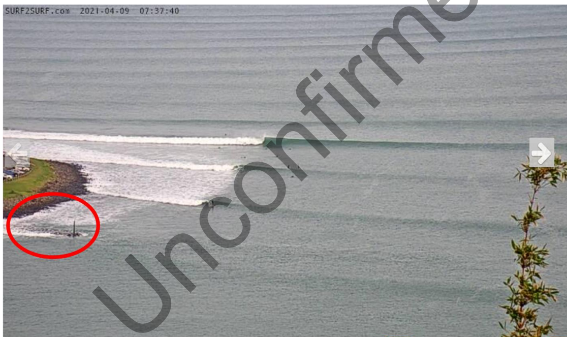
Figure 3: Overtopping of the breakwater structure 1hr before a neap high tide during moderate swell conditions observed on 9/04/21.
