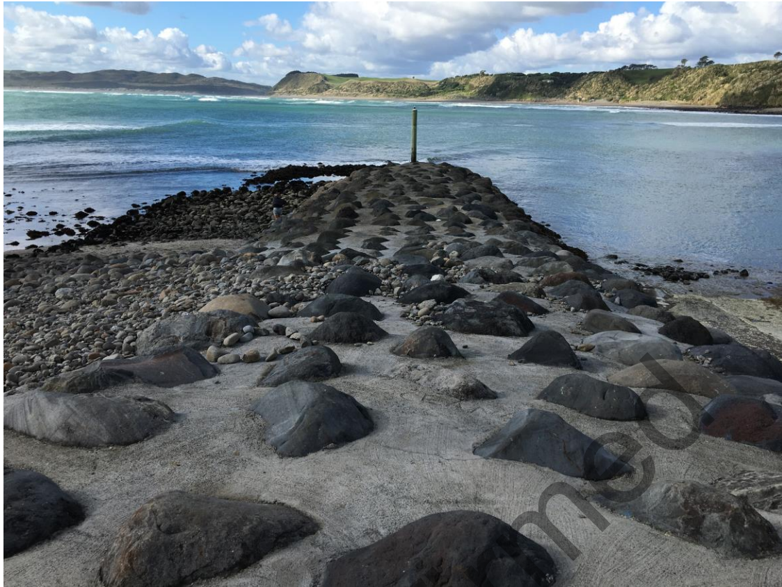
Figure 9: Photo showing the migration of rock material over the upper portion of the breakwater.
