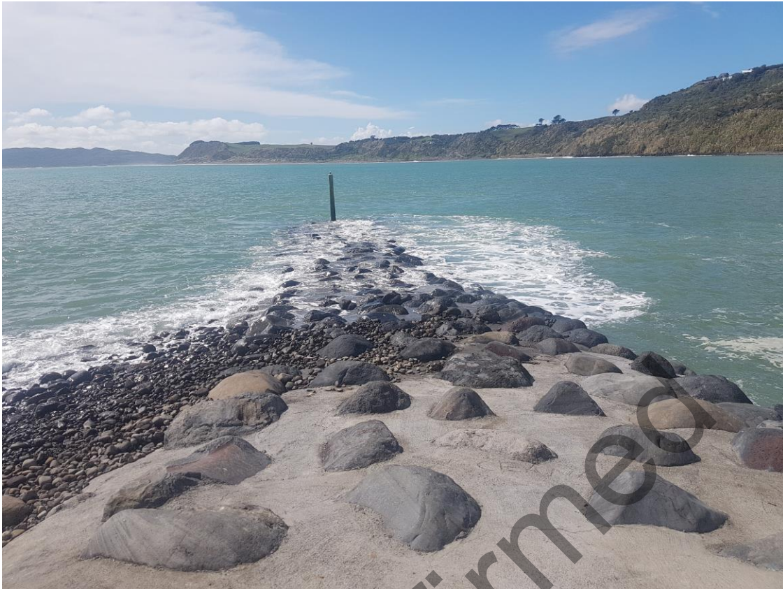
Figure 8: Wave overtopping event at the Manu Bay breakwater. Note the extent the white water line on the inside of the ramp indicating the dissipation of broken wave energy as the wave moves over the breakwater and into deeper water. The extent of wave penetration past the breakwater will be highly dependent upon swell conditions at the time.
