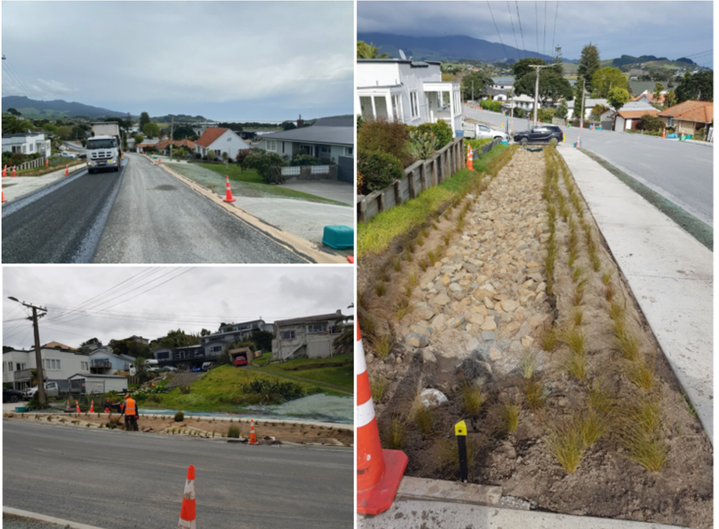
Looking south down Gilmour Street
