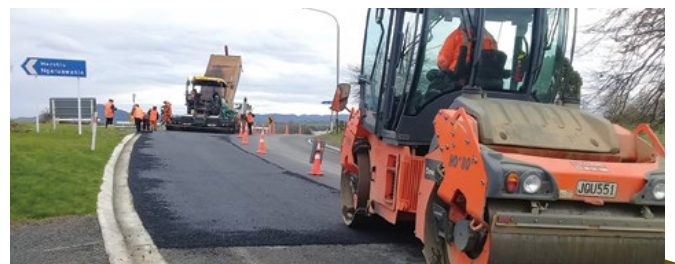
Beer bottle glass sand asphalt has been used for work on the Horsham Downs and Lake Road intersection.
