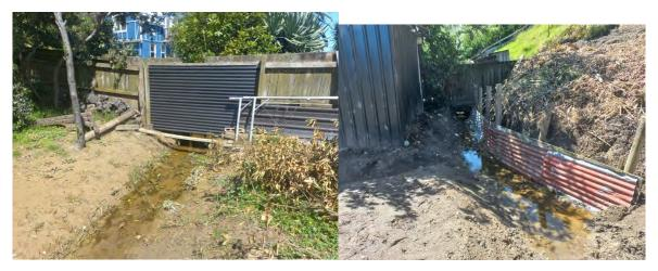
A contractor did maintenance works to remove the debris and reinstate the channel, allowing for the proper flow of stormwater. Temporary fencing was installed using available materials on-site to prevent soil erosion caused by rainfall.
