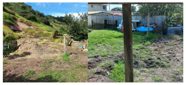
The two photos above show earth slips that completely blocked the existing open channel.
