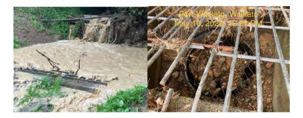
An overflowing issue occurred again on May 9, 2023. This is the second occurrence following the first one caused by Cyclone Gabriel in February 2023. Heavy debris and sediments rushed down to the Scruffy Dome asset, causing it to become blocked once again. WSL conducted cleaning work inside the manhole to ensure the flow of stormwater into the stormwater network.
