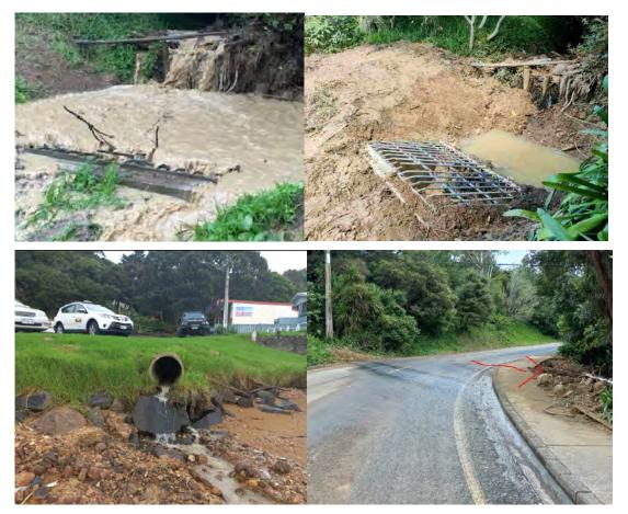
Immediately after the impact of Cyclone Gabriel, WDC/WSL assessed the damage situation and conducted necessary physical maintenance. The pipe connected to Scruffy Dome was thoroughly cleaned to ensure proper runoff from upstream to the outlet, as shown in the photo above.
