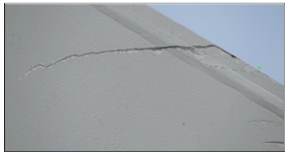
Paint damage on the bridge from contact during the building move.
