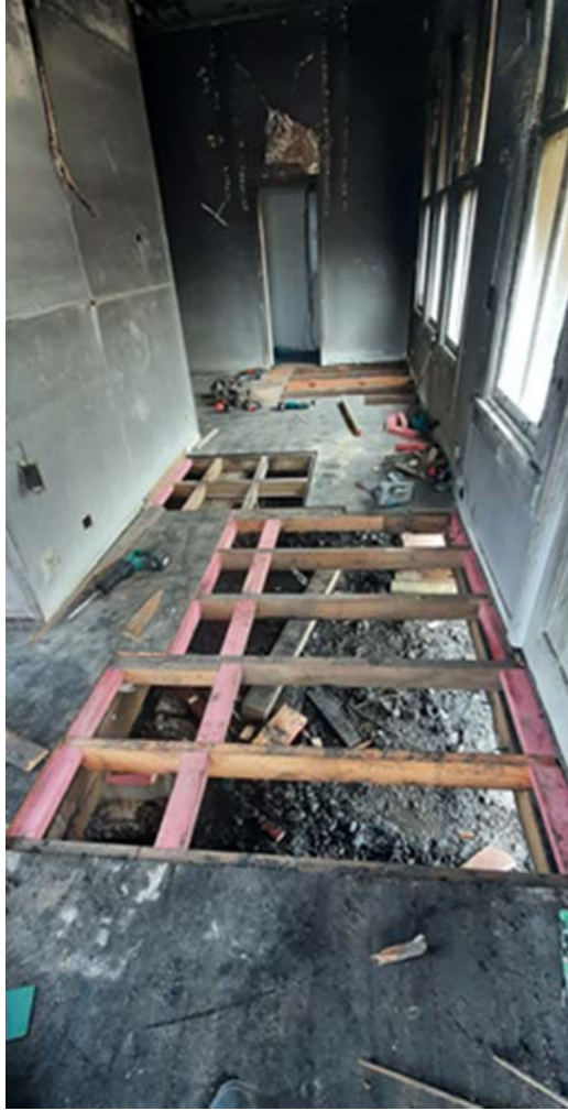
Interior repair where the temporary support barrels damaged the floor on collapse.
