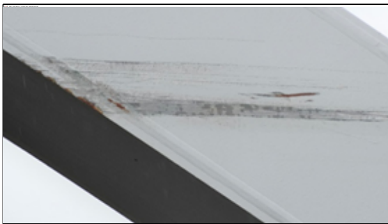
Paint damage on the bridge from contact during the building move.
