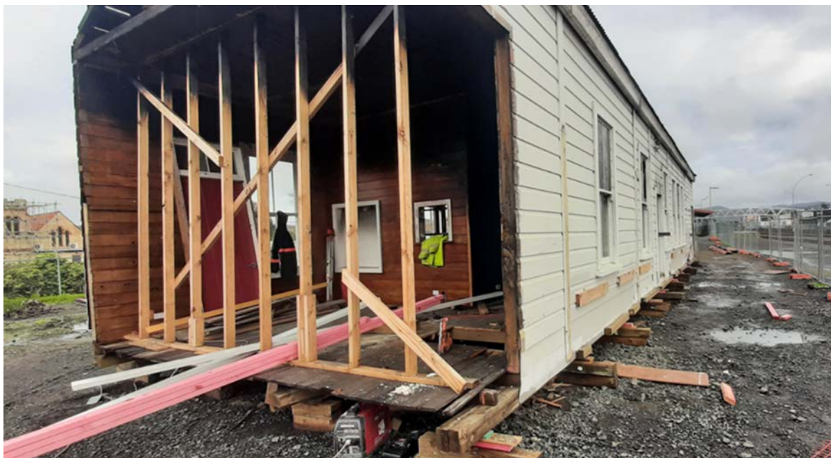
Damaged section with side awning removed and building levelled.
