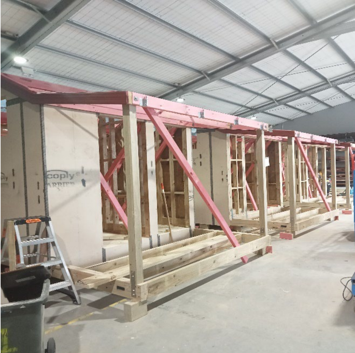
Toilet units being constructed in the Ngaruawahia factory.
