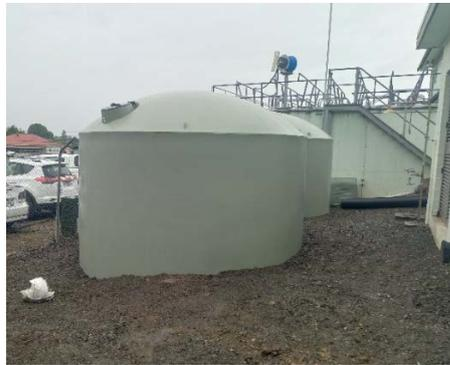
*The run to waste storage tanks were secured in position ready for the pipework to commence.*
