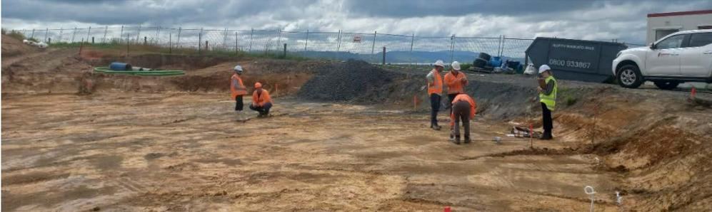
*Te Kauwhata – Reservoir 2 sub-base inspection ahead of the granular base installation*
