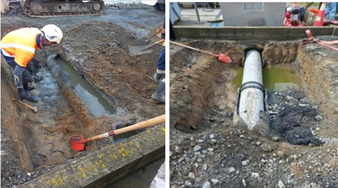
**Figure 2 - Corrosion at the treatment pond inlet (L) and temporary fix of a length of this pipe (R)**
