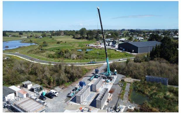
Te Kauwhata WWTP\_temporary Ultra filtration plant has been installed and commissioned by Spartan/Veolia and is now operational. Initial 2 test results show an improved treatment performance for suspended solids from >30g/m3 to 3g/m3 and then 1.6g/m3 against a measure of 15g/m3, which is a great result.
