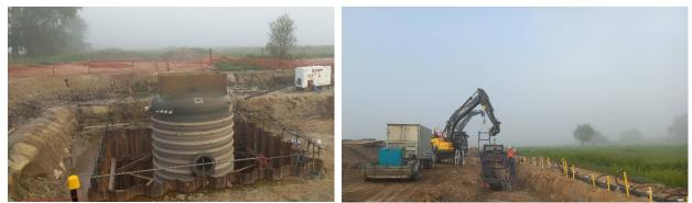
*Ngāruawāhia Pipeline – The wet-well construction and the pipeline are both well underway.*
