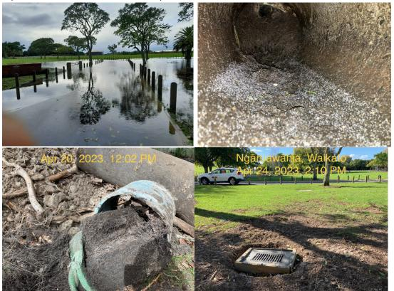
A significant line fault was repaired at Marine Parade PS, Raglan. This fault was identified via the CCTV surveys carried out in the area. The roof of the 150mm line had completely degraded, so the replacement of approximately 6m of the line was required.
