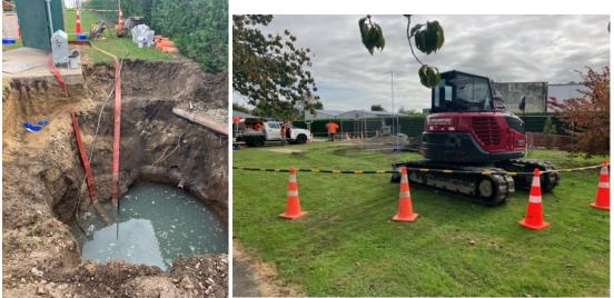
A sewer line fault was repaired at Camp Ground PS in Raglan. Manhole inspections carried out by field staff identified a manhole chamber with severe root intrusion. Root cutting and CCTV was carried out, and the CCTV identified further issues on the 100mm line approximately 1m from the chamber. The line sat 2m deep, so trench shields and a large digger was required to excavate down.
