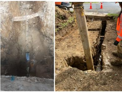
The Good Street pump station in Matangi had a wetwell replacement due to I&I issues experienced at the plant. The well had a degraded base allowing for ingress to occur.
