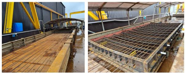
Te Kauwhata – Reservoir 1 - Fabrication of the prestressed concrete wall panels
