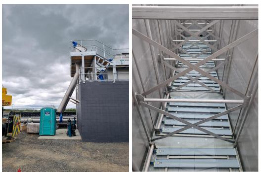
Te Kauwhata WWTP - New inlet screens and an Aerostrip® diffuser grid
