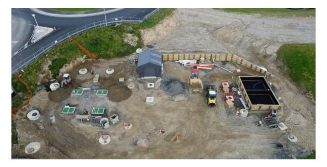
Upgrade the Horotiu wastewater network to accommodate growth in the catchment to maintain a reliable, safe and efficient wastewater network. The pump station is nearly complete. A connecting gravity sewer and rising main in the new road is being built by WDC.
