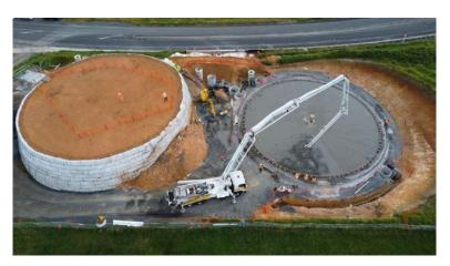
This project replaces the existing Te Kauwhata Reservoir with a 1,500m3 reservoir to maintain a reliable and efficient water supply network. The reservoir construction is well underway and on track to complete in 2023.
