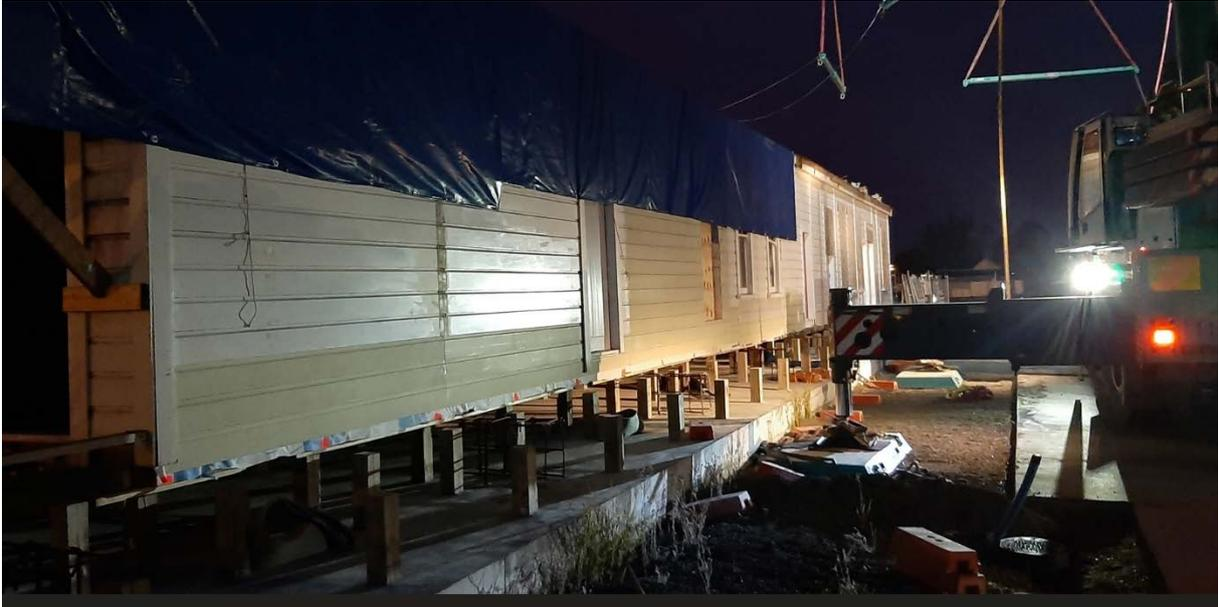
*Damaged section being placed on piles in permanent location.*
