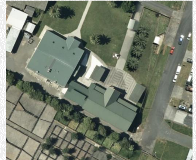
BEFORE INSTALLATION • Site without solar panels
