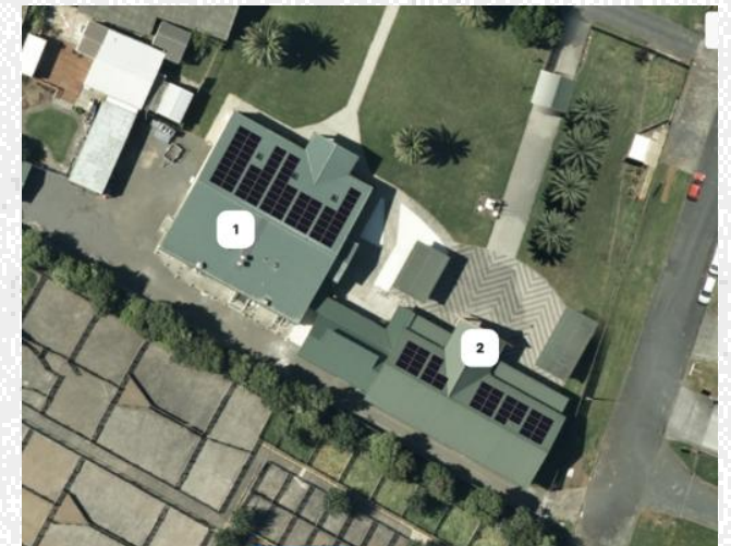
AFTER INSTALLATION • Site with solar panels
