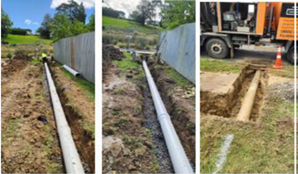
Critical Damaged 50m Pipe Replacements in Te Whereo Crescent – Meremere
