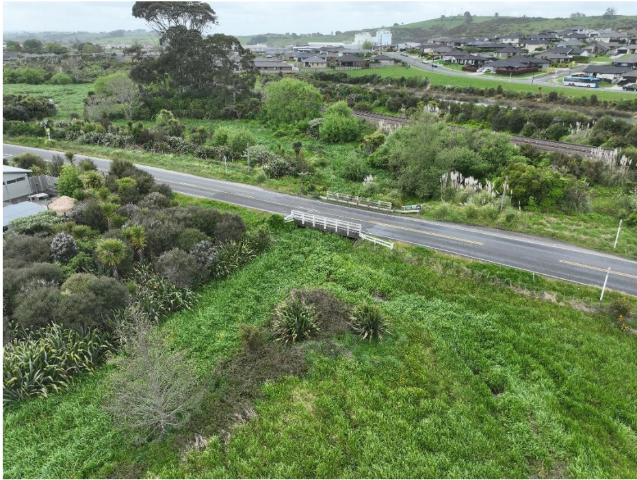
Aerial view of Pokeno Rd vehicle bridge looking south
