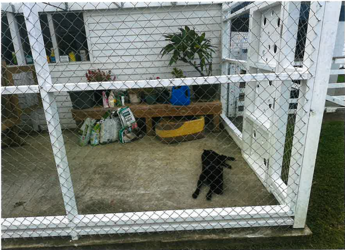
Completed Containment Area 1
