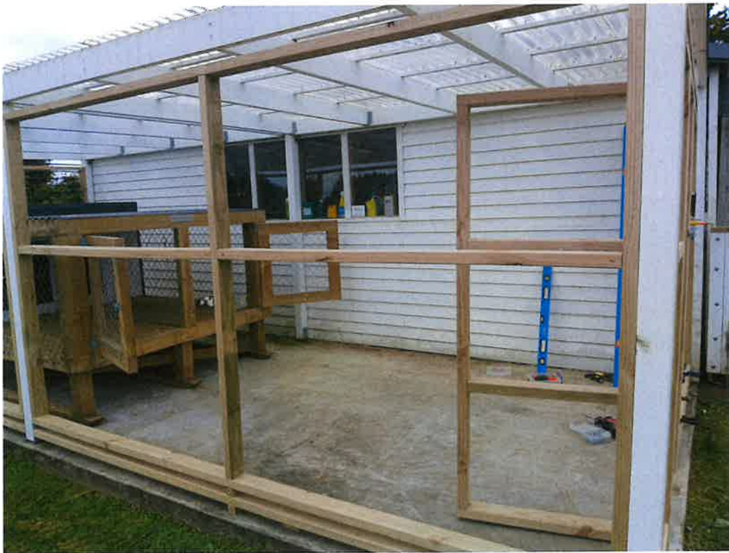
Enclosure being built including kennels
