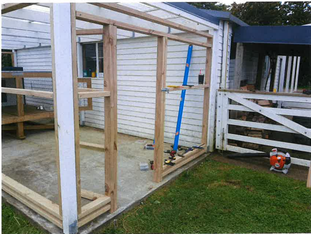
Enclosure being built
