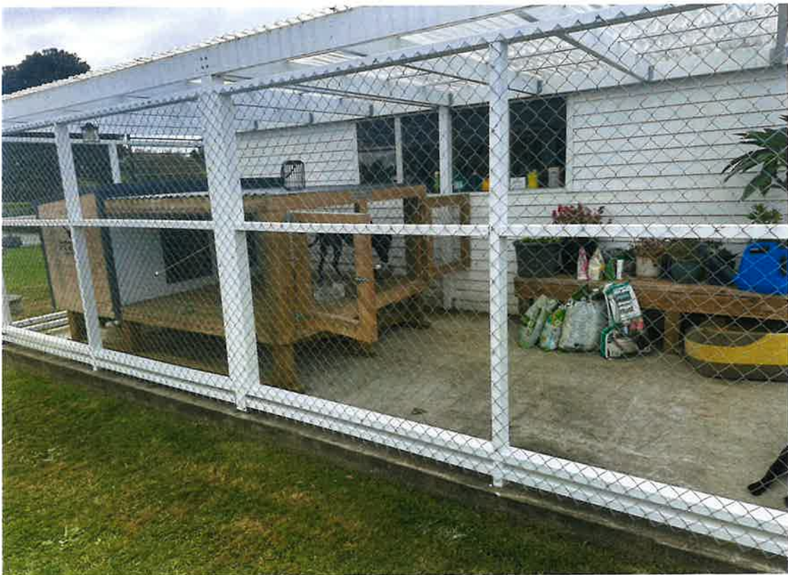
Completed Containment Area 2
