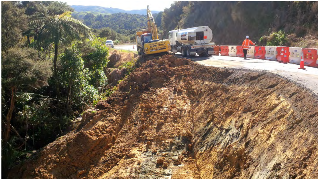
Picture 1: Slip repair at Ohautira Road
