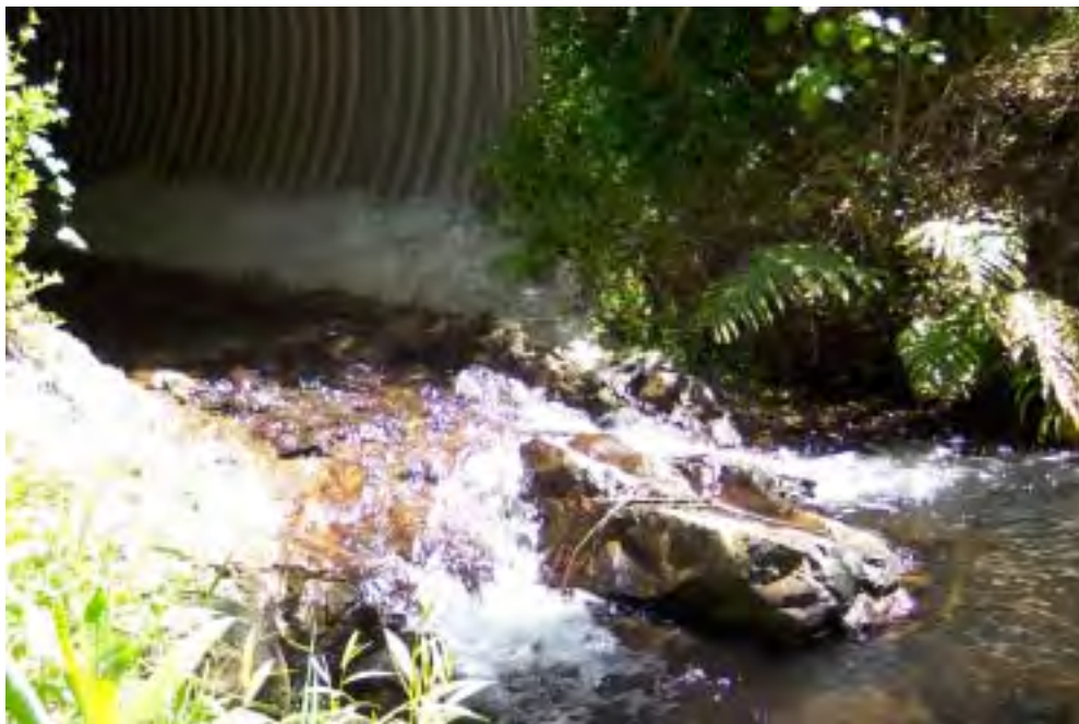
Figure 15: Rock rubble has been placed at the end of culverts so native fish can migrate past these structures.
