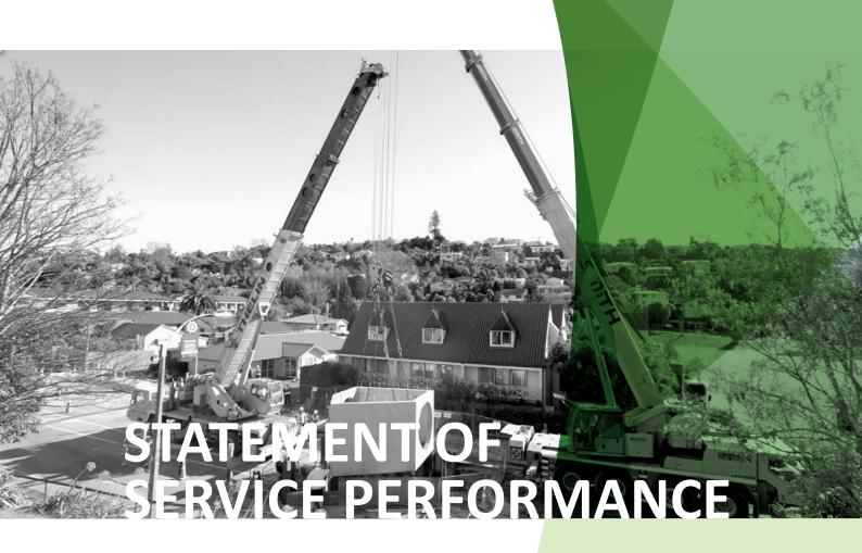
A stormwater mixing chamber is lowered into place as part of a comprehensive upgrade on the Little Go Stream. Nelson City Council.
