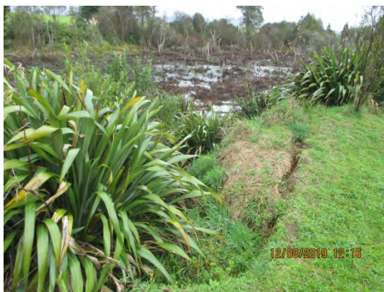
Slumping of existing track outside of Lot 20
