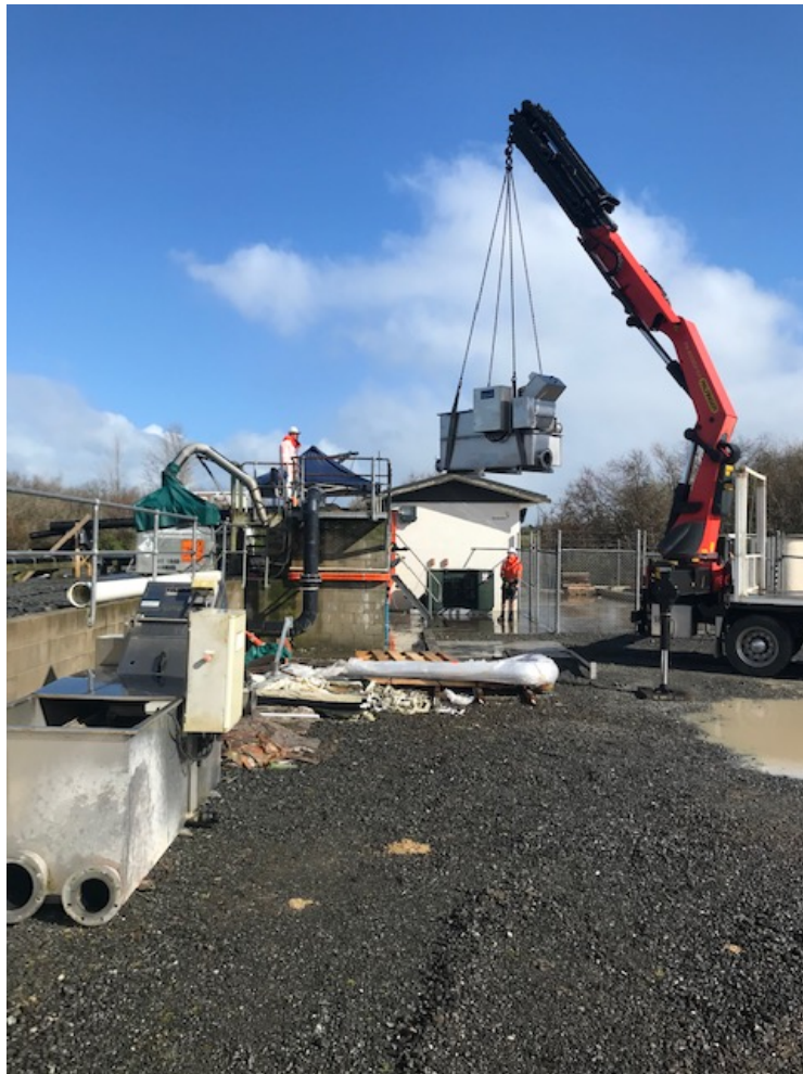
Step screen installation
