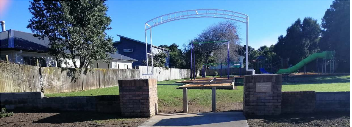
Warihi Park entrance upgrade to allow maintenance vehicle access
