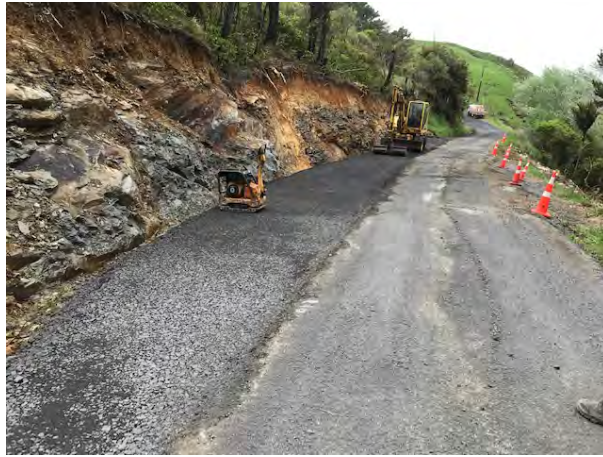
Wairamarama-Onewhero Road slip repair
