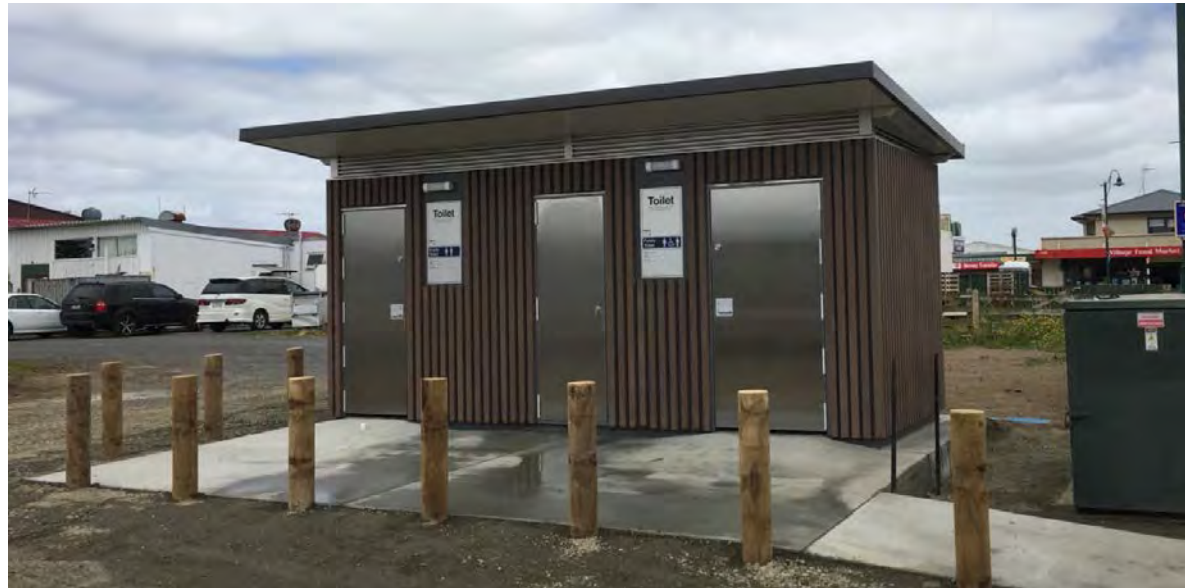
Completed toilets at St Stephens Ave, Tuakau
