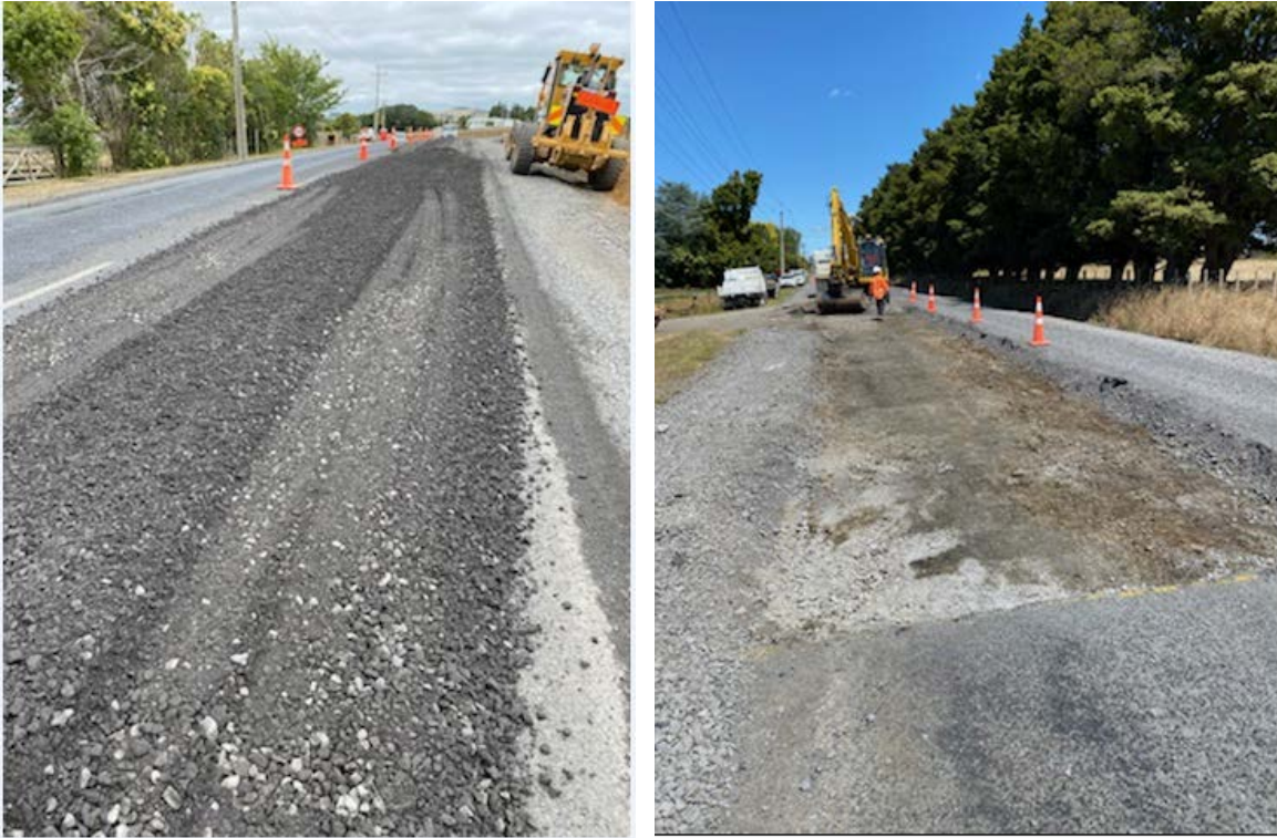
Mercer Ferry Road Progressing
