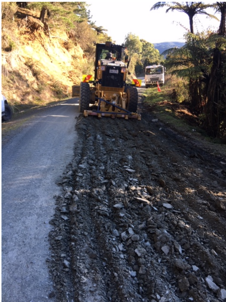
Reshaping on Otoroha Trig Road
