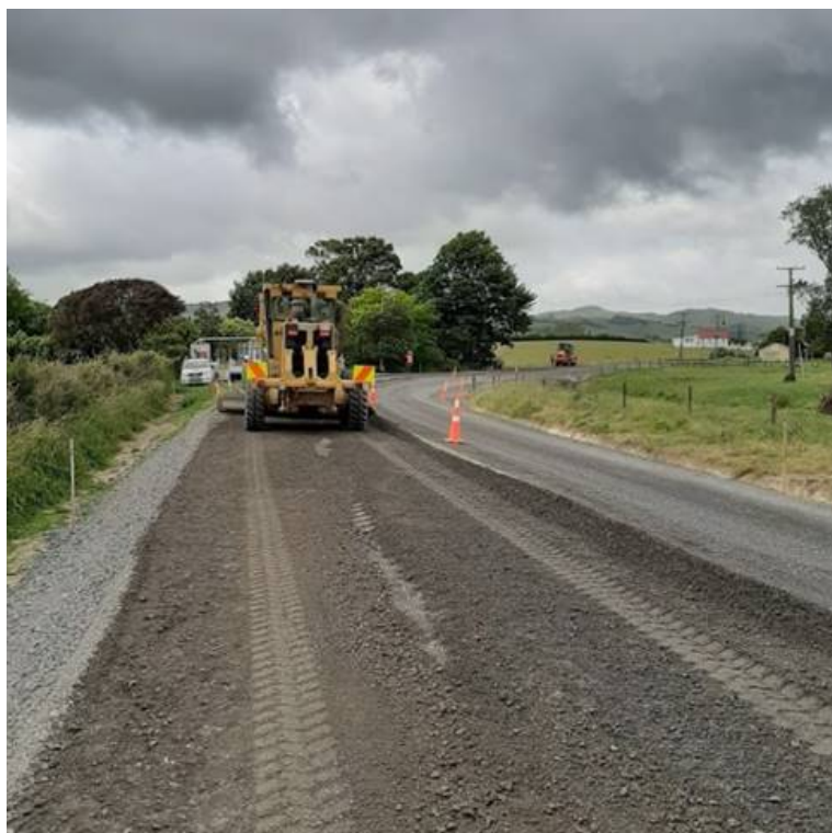
Taniwha Road Second Half Progressing
