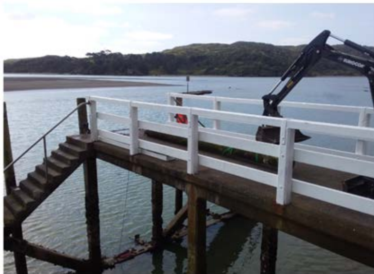
Fender Pole Replacement Underway
