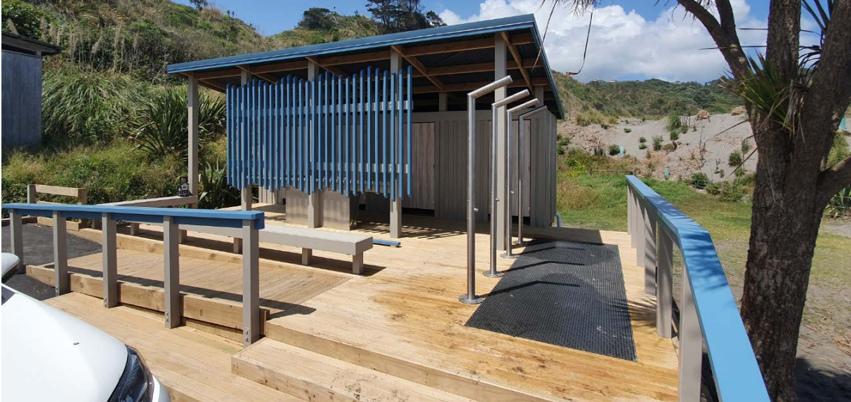
Completed toilet and outdoor shower facilities.
