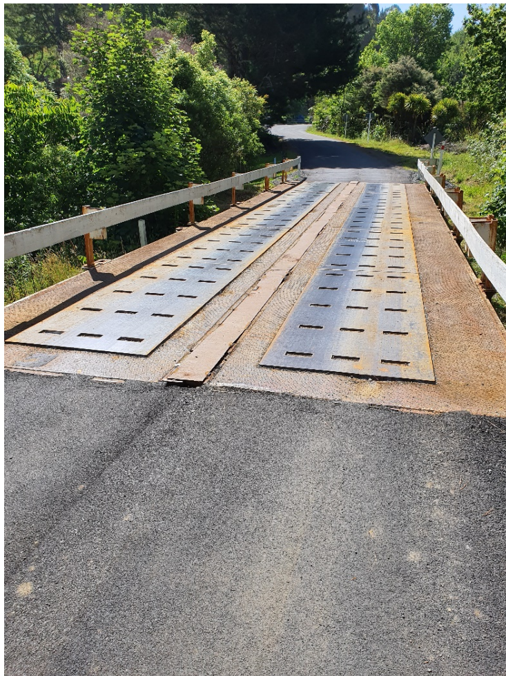
Otonga Valley Road Bridge Deck Re-skinning
