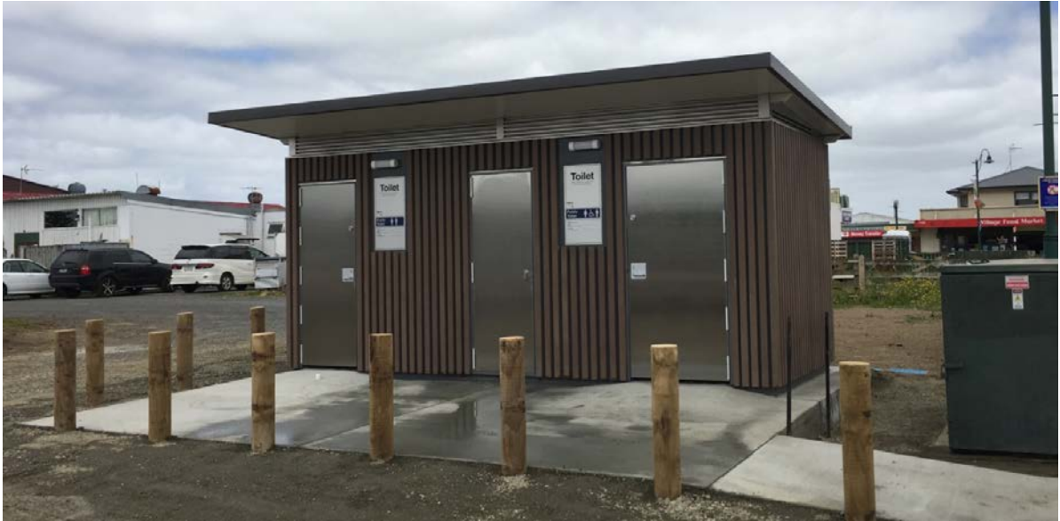
Completed toilets at St Stephens Ave, Tuakau
