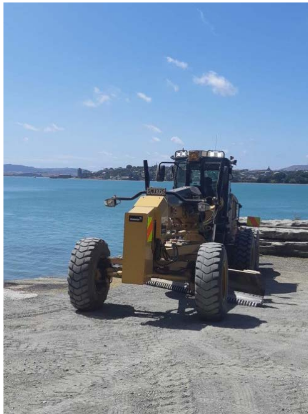
Grader at Te Akau Wharf Road
