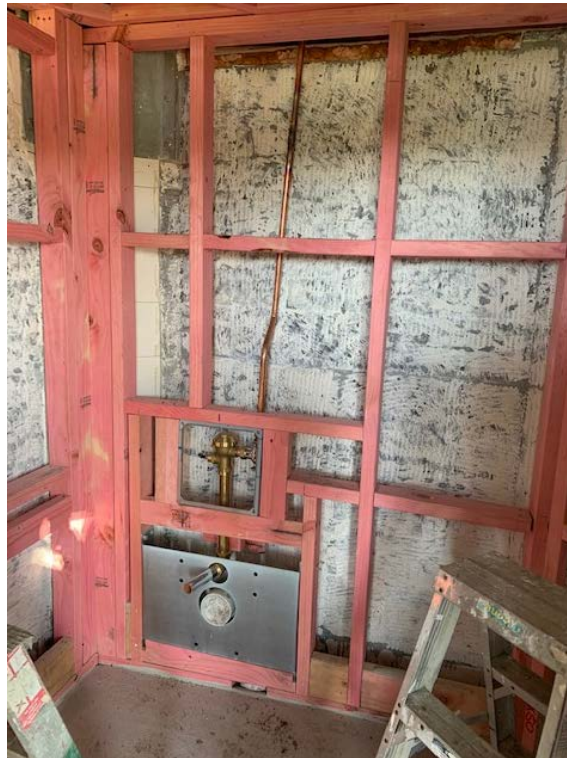
The Point, Ngaruawahia toilet refurbishment
