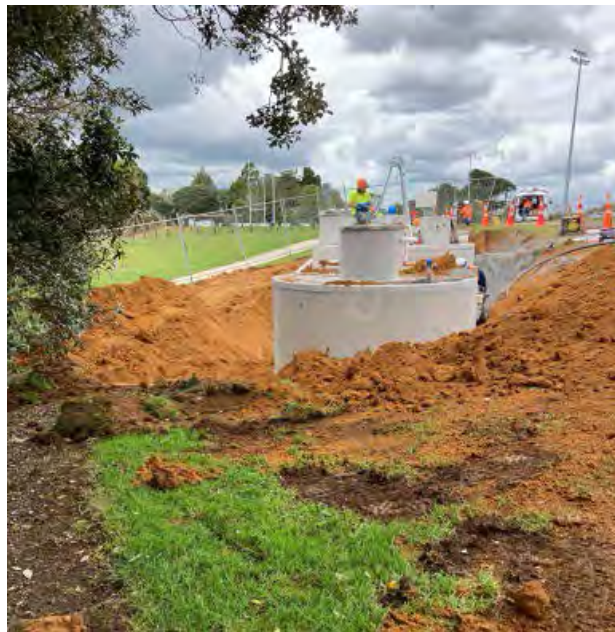
Installation of additional tanks
