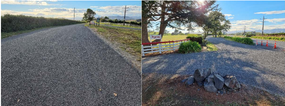
New sealed surface
