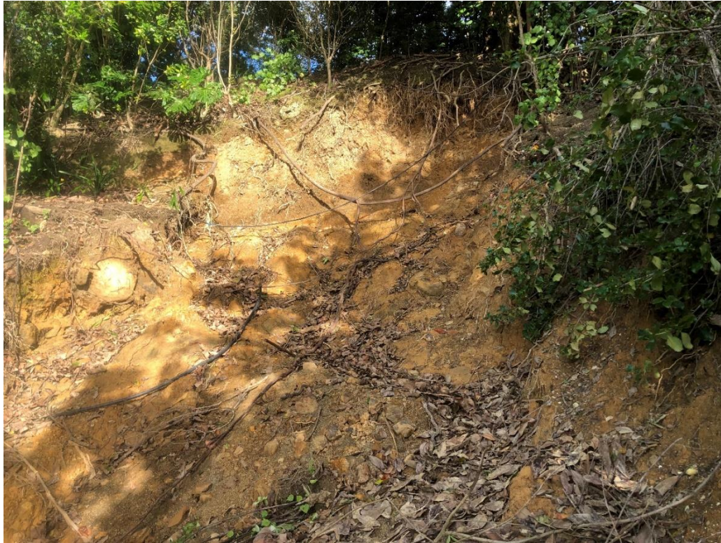
Photograph 13: Landslide within [REDACTED]
