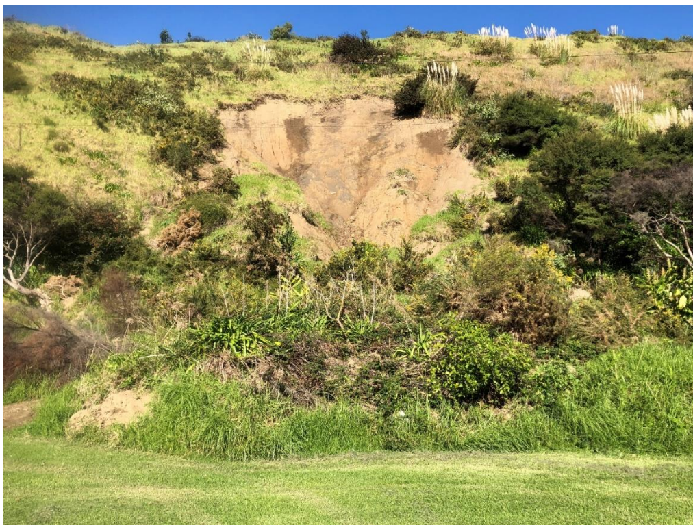
Photograph 12: [REDACTED] Large Landslide 19
