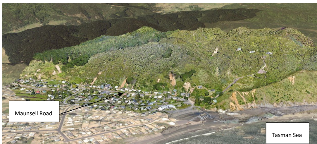
Figure 2.2: Aerial photograph looking south-east towards Maunsell Road.
