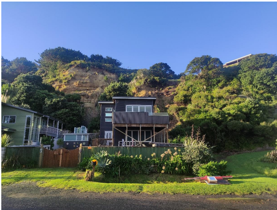
Photograph 4: View of Landslide 1 & 4 [REDACTED]
