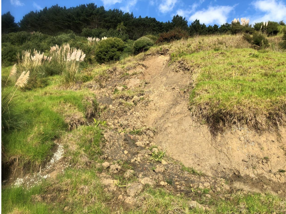
Photograph 9: View of Landslide 13
