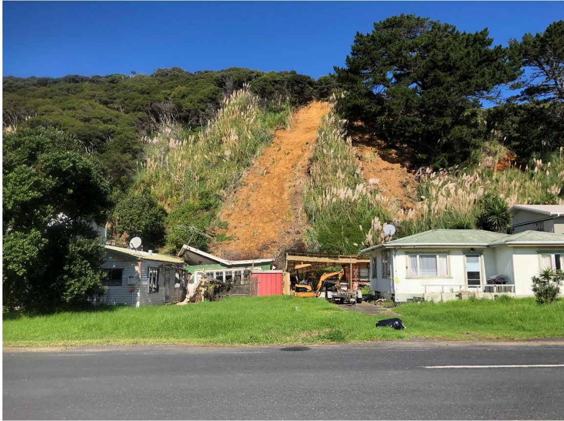
Photograph 7: View of landslide 9
