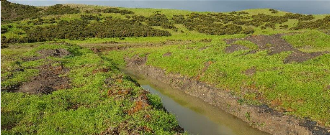
Figure 2: Main channel from pond. Seed and mulch stockpiles. Install rock check dams and hydroseed batters.
