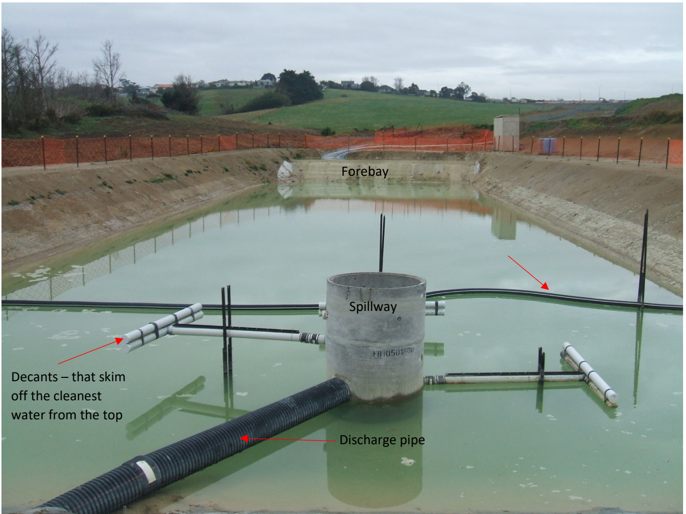
Example of a sediment retention pond (photo courtesy of Southern Skies Environmental – Erosion & Sediment Control Specialists working with Gleeson)
