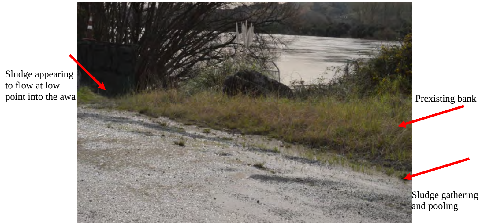
Photograph showing water laden with silt flowing directly into the awa
