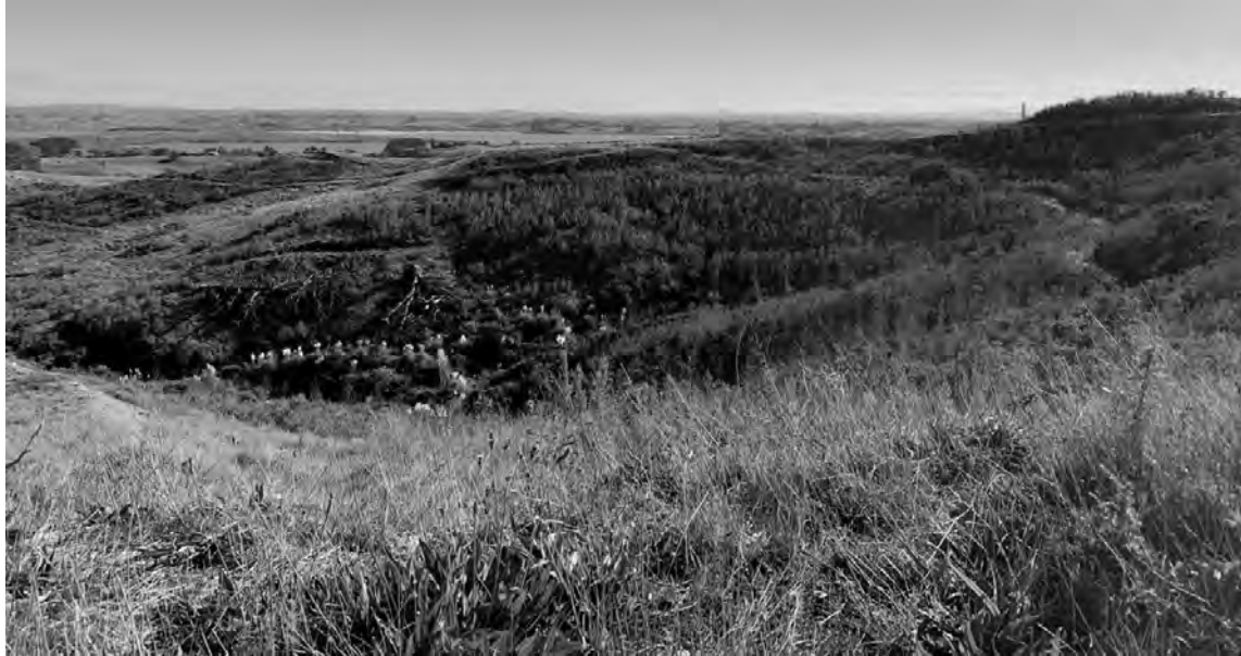
Photo 1: Fill Area 2 looking north west
