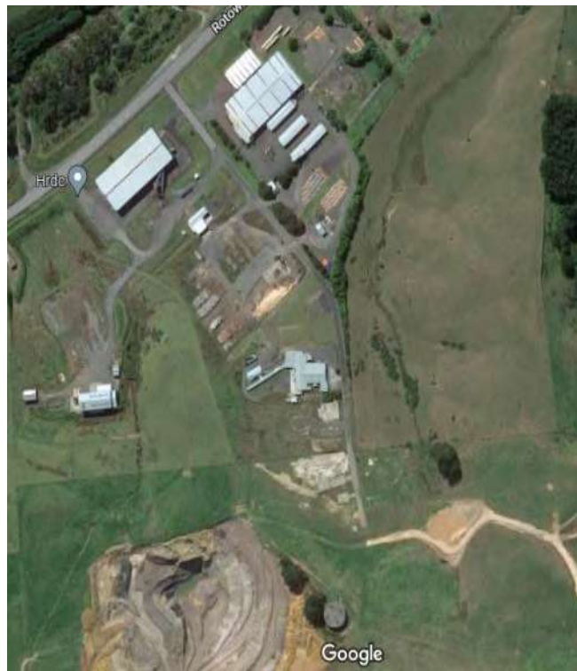
Close up of the access road through the heavy industrial zone.
