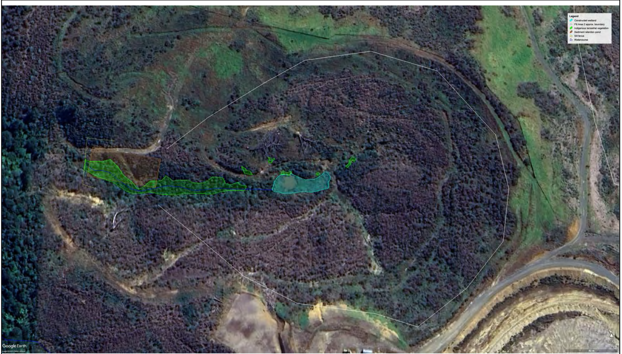
Fill Area 2 showing works footprint, constructed wetland and areas of indigenous terrestrial vegetation.
