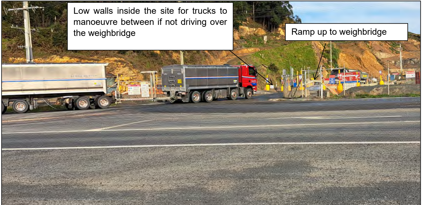
Figure 5: Existing vehicle crossing to the Quarry site (20 June 2022)
