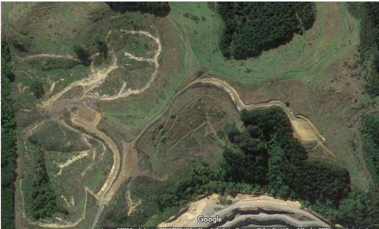
Tracks and other vegetation free areas on the northern side of the property outside of the quarry pit
