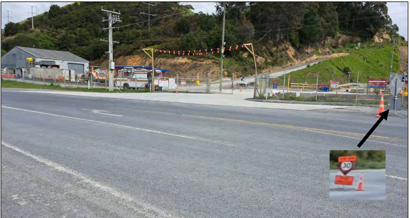
Figure 6: Existing vehicle crossing has recently been upgraded to concrete. Note the temporary speed limit and road sweeper sign (8 October 2022)
