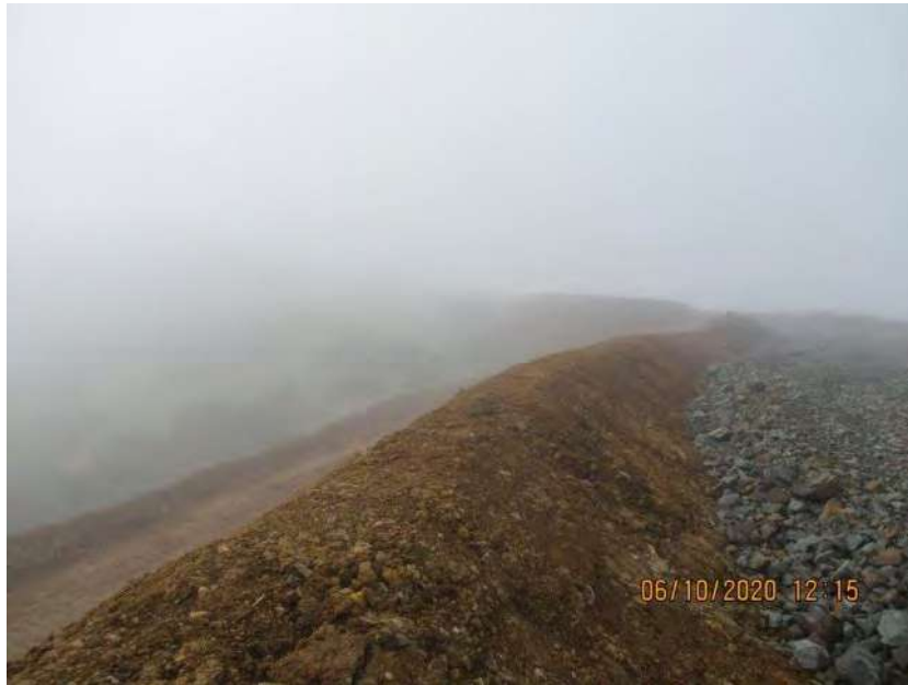
Photograph supplied of inspection, with fog impeding the ability to see
