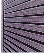
4. Half Eurotray Roofing
