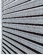
4. Half Eurotray Roofing
