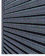
4. Half Eurotray Roofing
