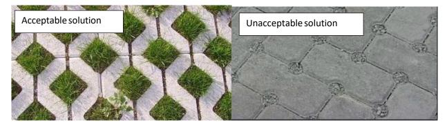
Figure 1: Pervious pavement acceptable and unacceptable options
