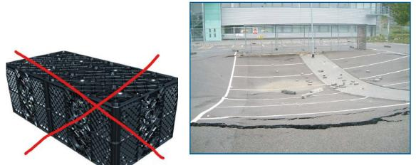
Example of the consequences of failure of a modular geocellular tank after three years
