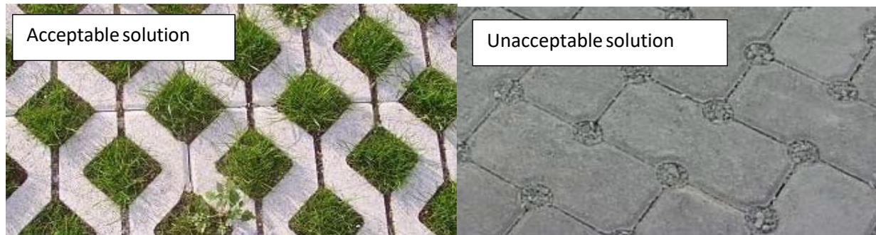
Figure 1: Pervious pavement acceptable and unacceptable options
