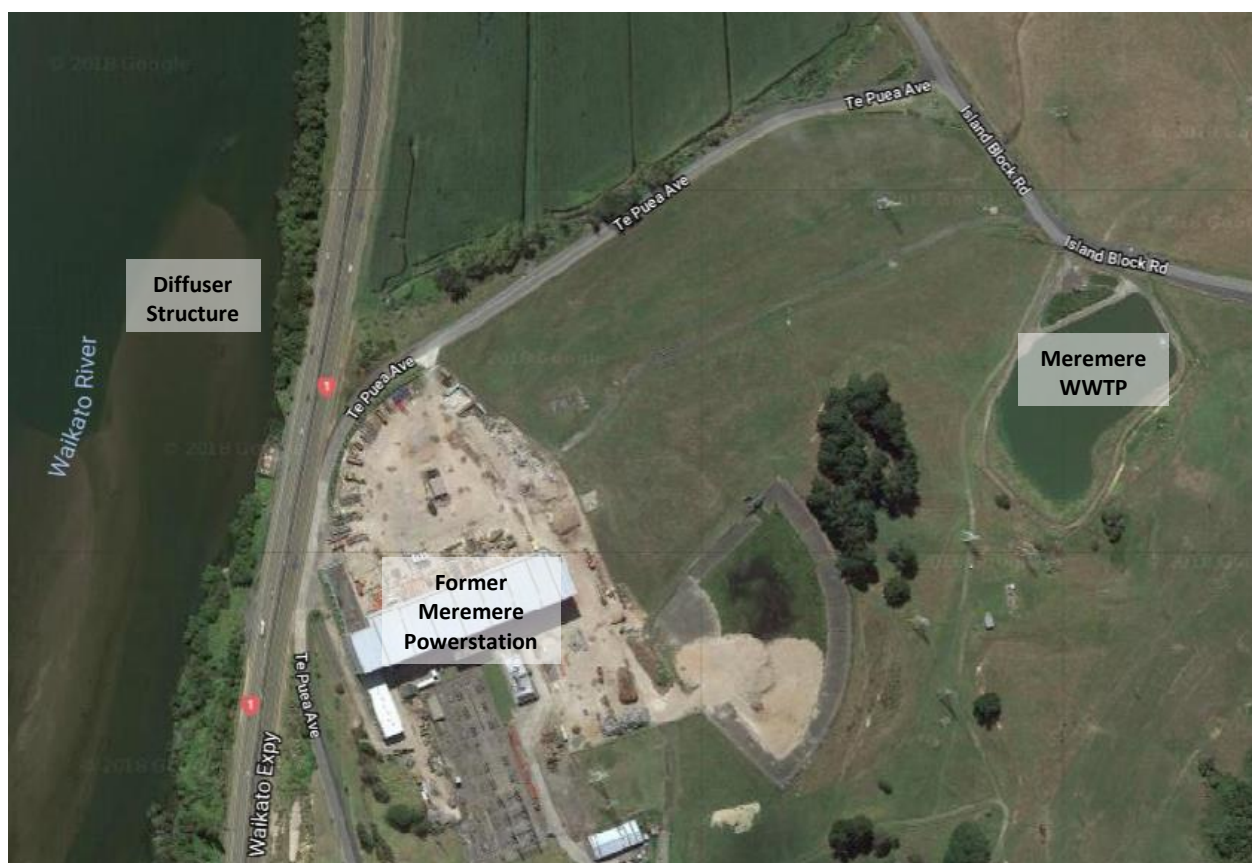
Figure 1: Location of Meremere wastewater treatment plant
