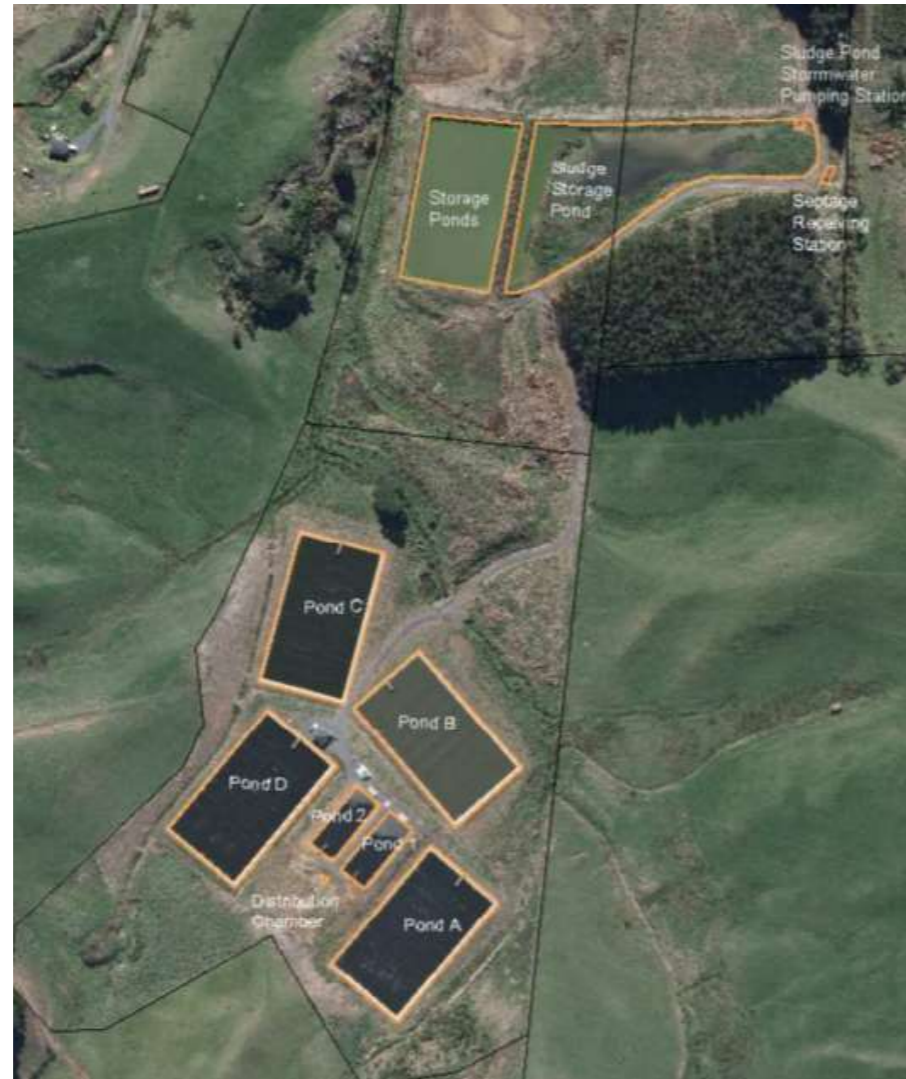
Figure 1: Raglan WWTP overview
