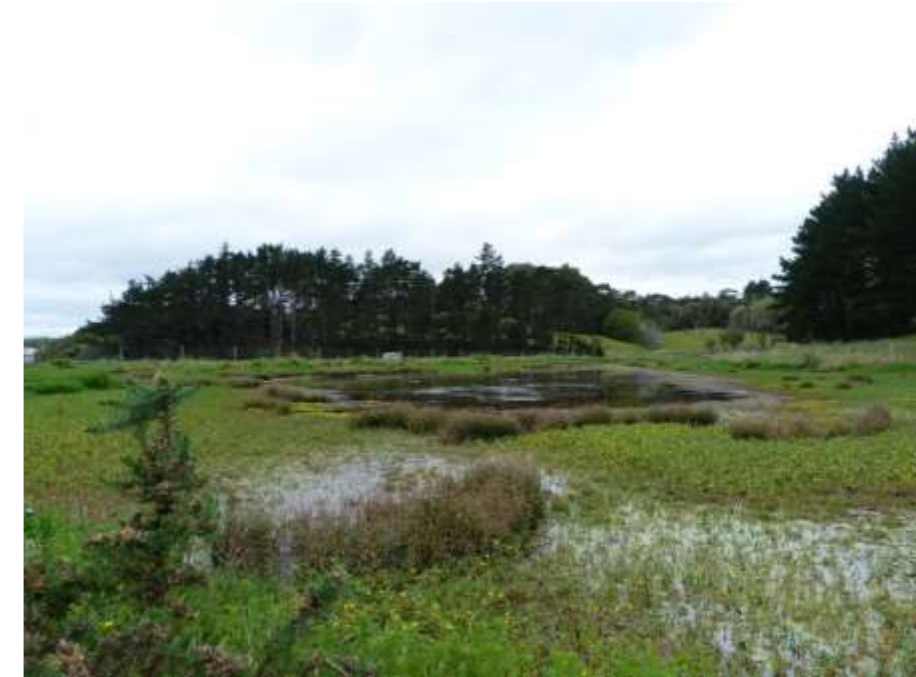
Figure 2: Raglan WWTP sludge storage lagoon
