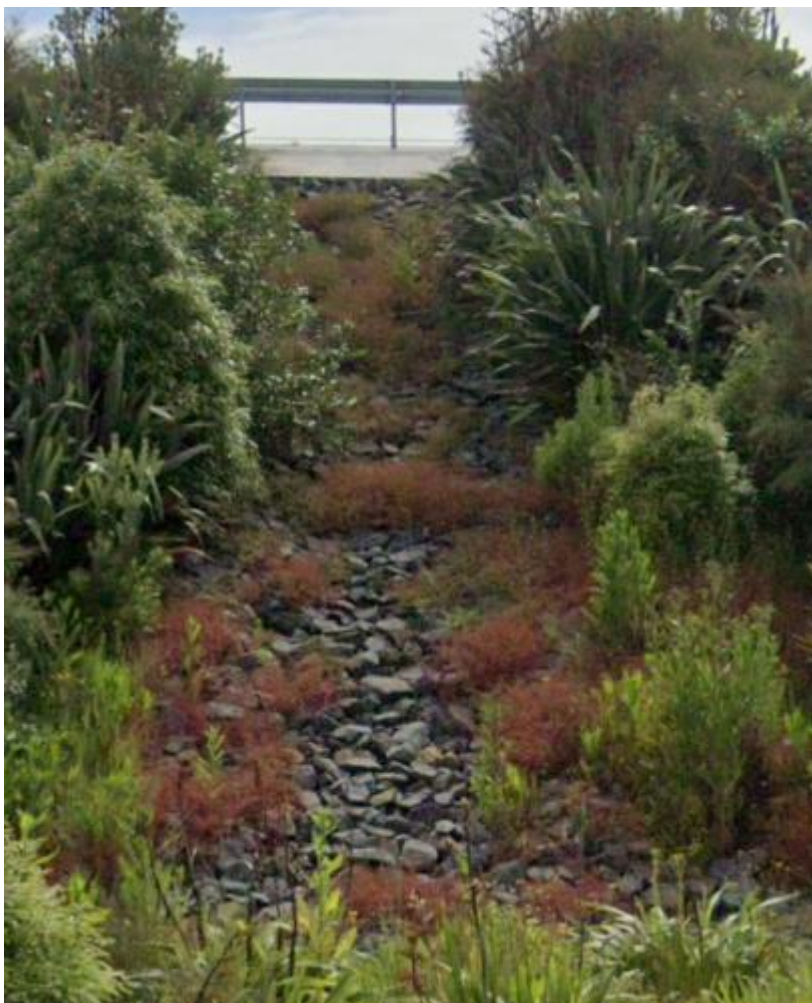
Figure 6 - Example of rock channel on slope
