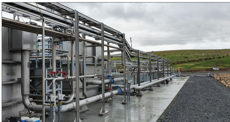
Meremere wastewater treatment plant membrane aerated biofilm reactor unit.
