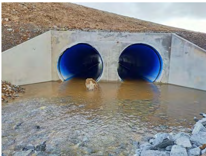
Figure 34 Whitikahu Road Culvert Replacement
