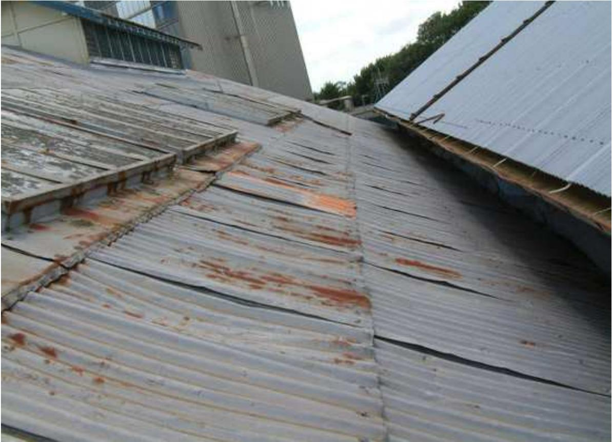
**Corrugated iron on roof is in poor condition.**
