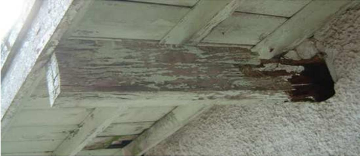
**Rotting beam from water getting under corrugated roofing.**
