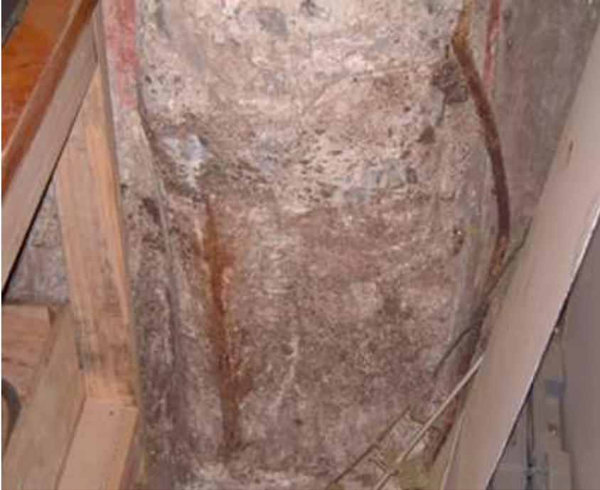
**Pillars scraped away by front end loader, exposing reinforcing.**
