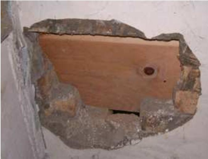
**Holes in walls where front end loader has run into walls, holes have been simply boarded up from the other side of the wall to cover the holes.**
