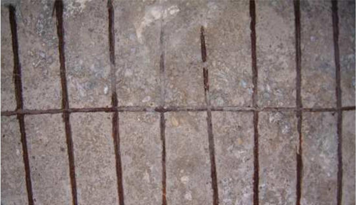
**Shot of roof showing rusted structural steel**
