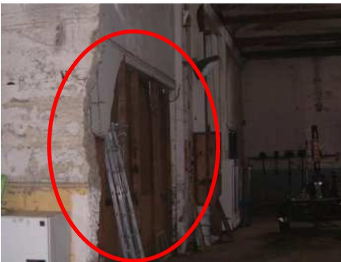
**Hole cut in wall adjacent to hole with structural column hanging down.**
