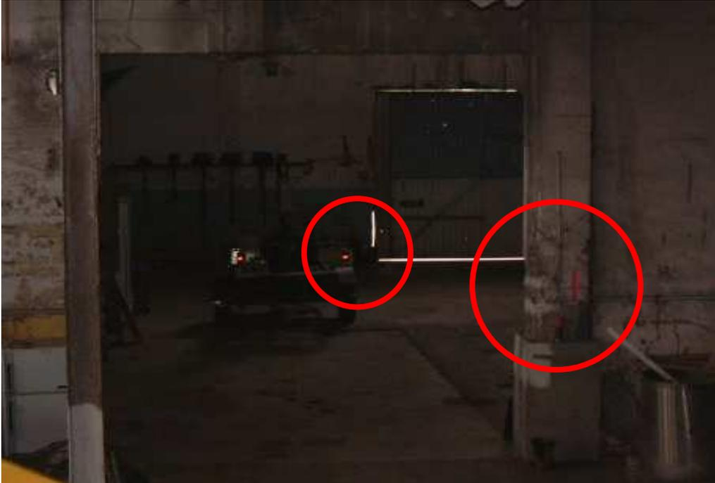
**Hole in wall with structural column hanging. Damaged columns circled**
