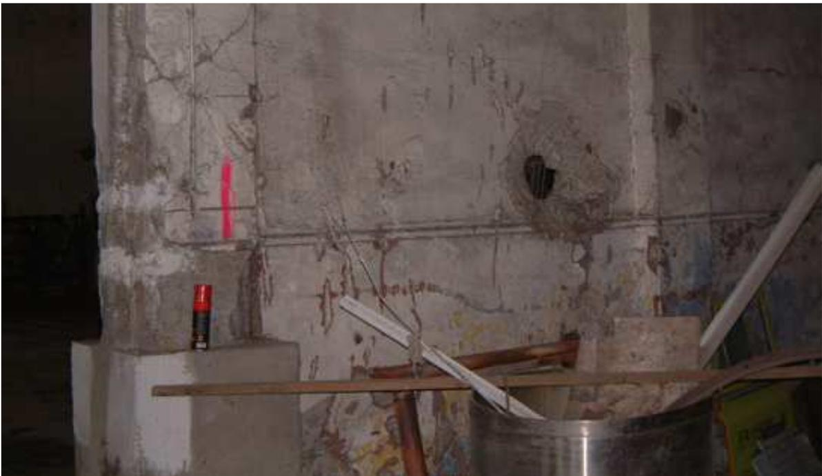
**Close up showing holes in wall and damage by front end loader.**
