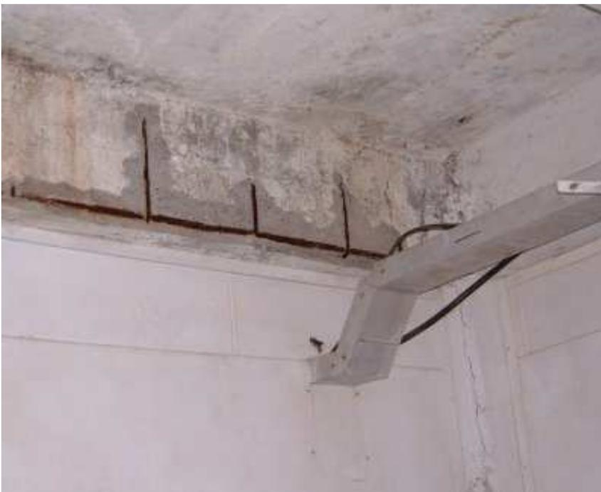
**Shot of roof showing rusted structural steel**
