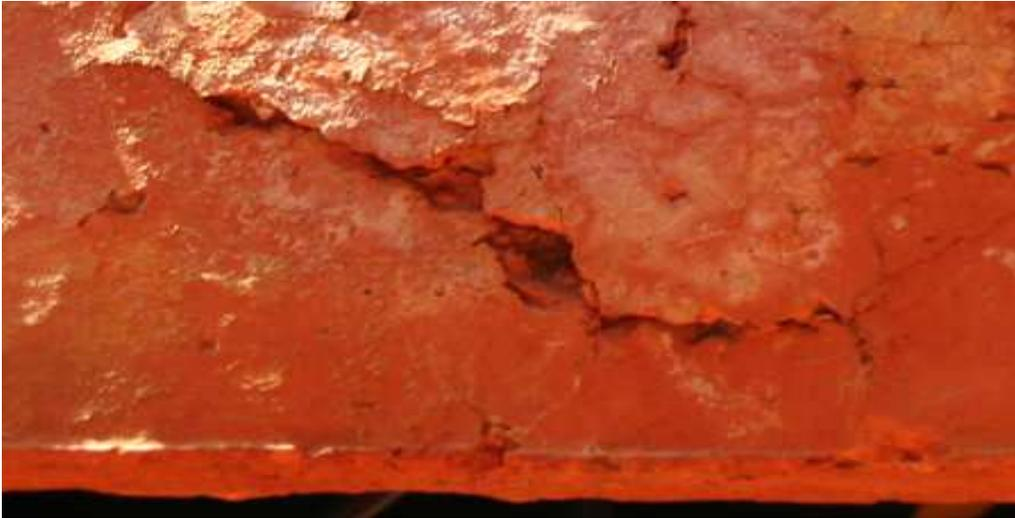
Bottom face of tile blown from water freezing the inside of the tile and expanding.
