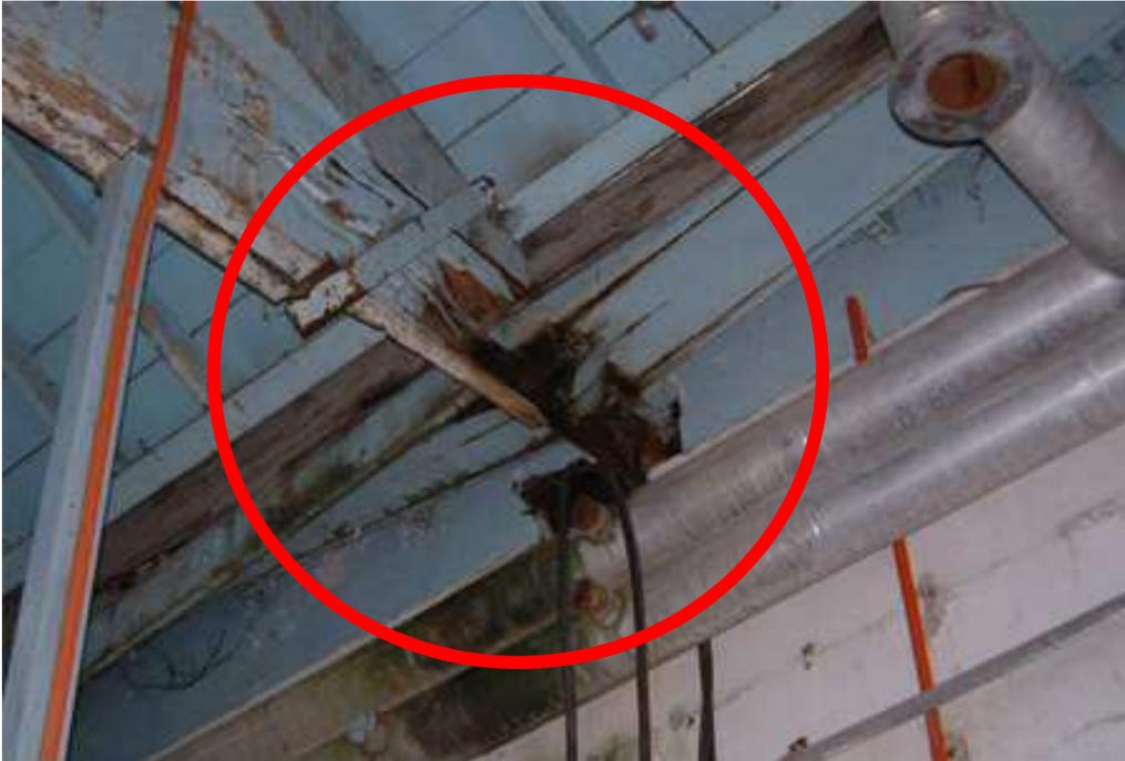
**Leaking internal gutter, rotting trusses.**
