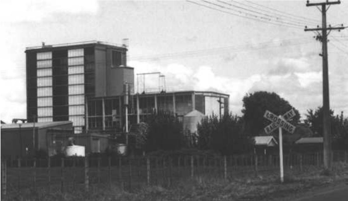
**Spray dryer to the left and 5-effect evaporators in the lower building on the right, photo 1985.**
