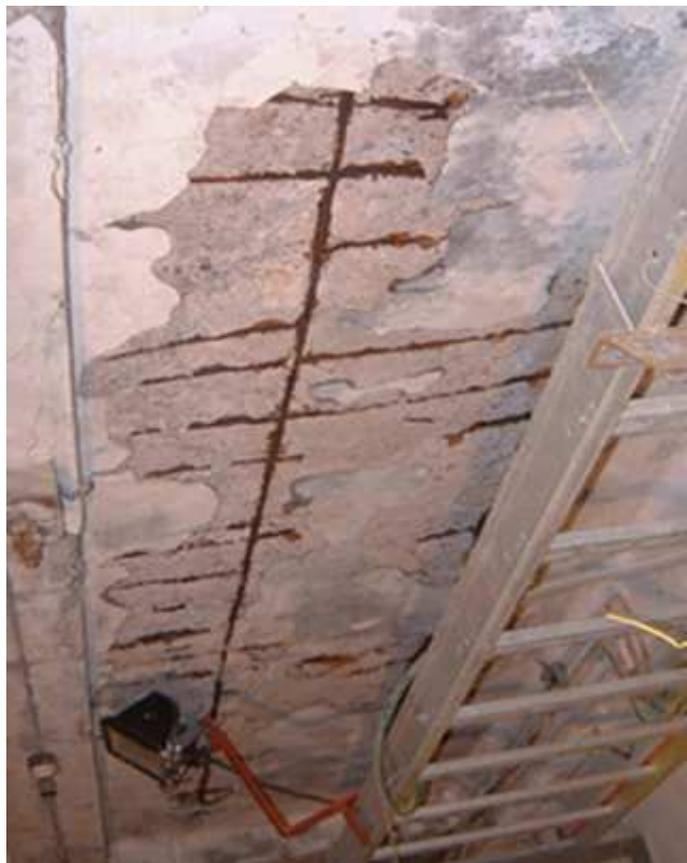
**Structural steel rusting and blowing concrete.**
